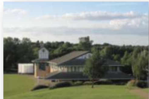
Figure 9: Campbell Park Pavilion
